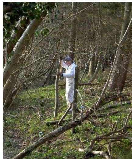
Driving in a fence post
